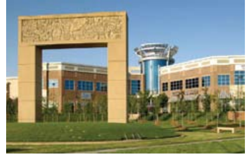
The south-west corner of Johnston Road (521) and Ballantyne Commons Parkway.
